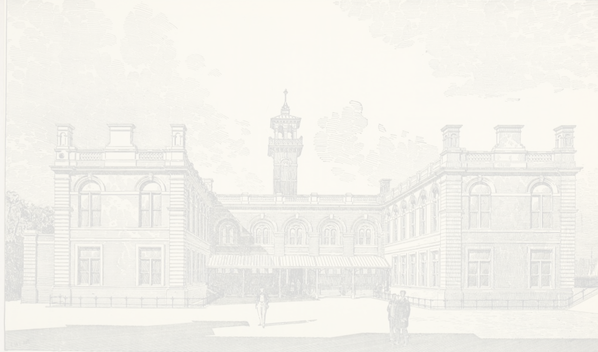
MEDICAL SCHOOL, WITH RECENT ADDITIONS. NORTH VIEW.
